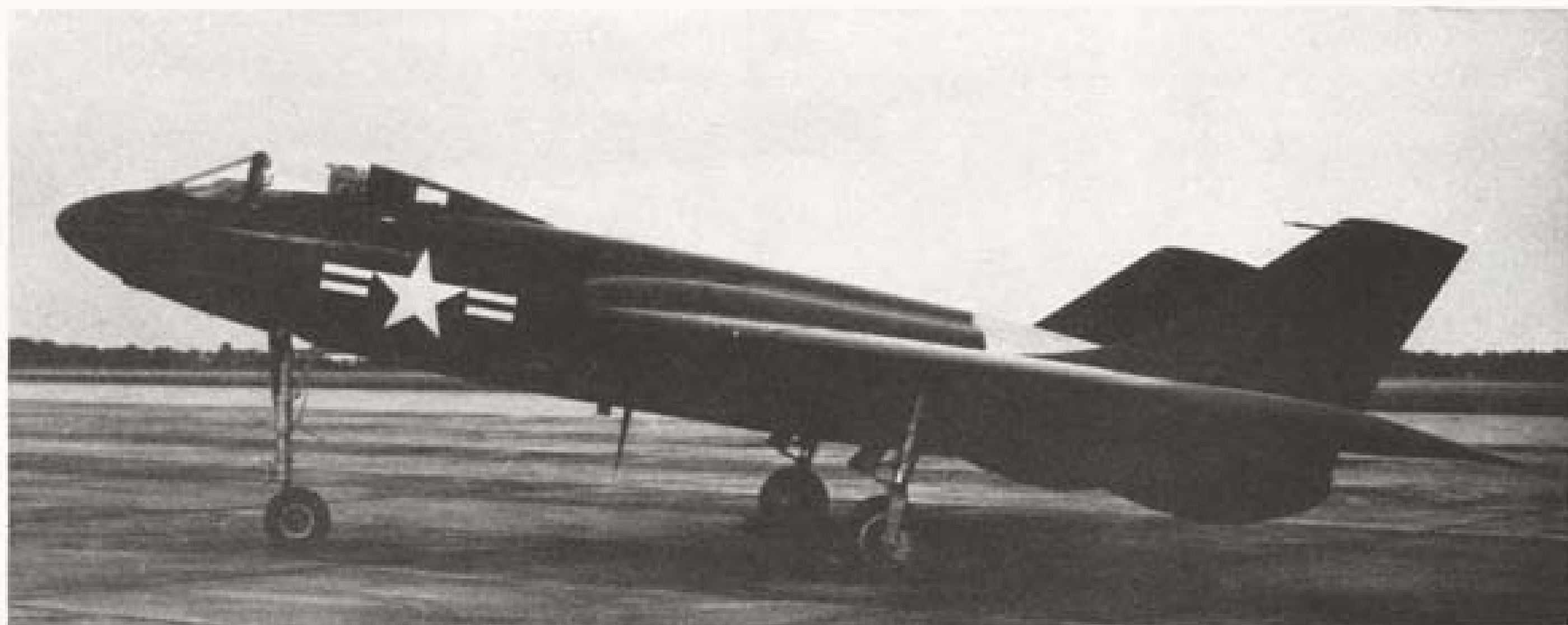
The CHANCE VOUGHT CUTLASS F7U is a tailless swept-wing carrier based single-seat jet fighter.
