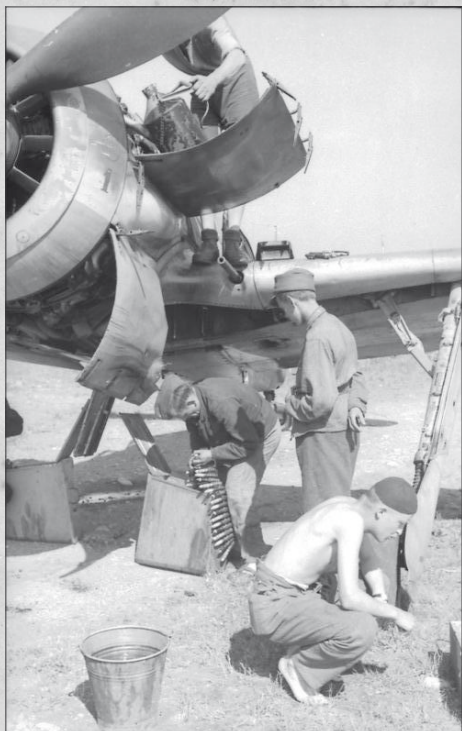
Finnish soldiers helping to load 20 mm ammo for Fw 190 A-6 „white 4“. Note the small number „1“ on the engine cowling, which suggests, that the engine possibly came from another plane.
